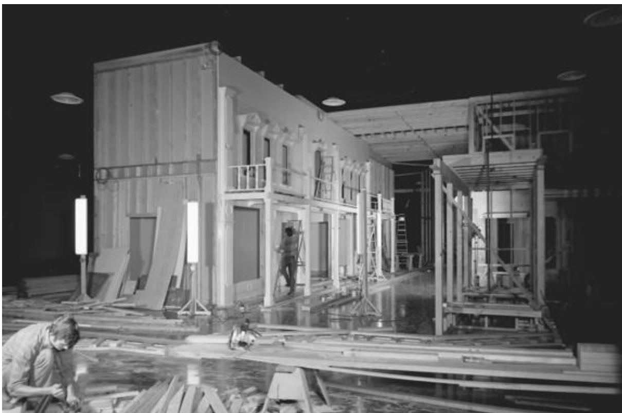
Figure 5. Scaffolding for Old Town. The building on the left is the Grand Hotel, with the parlour in its bottom storey (c. 1970). 69
