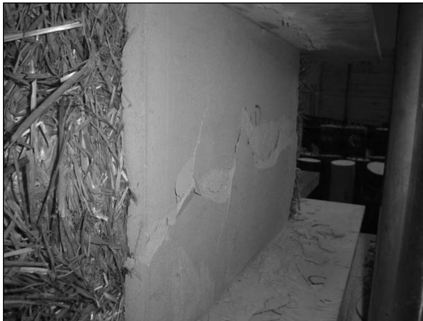
Figure D.3: Typical Failure of an On-Edge Plastered Straw Bale
