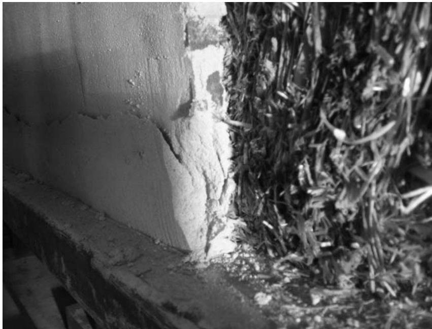
Figure 6.17b: Failure of Specimen C12
