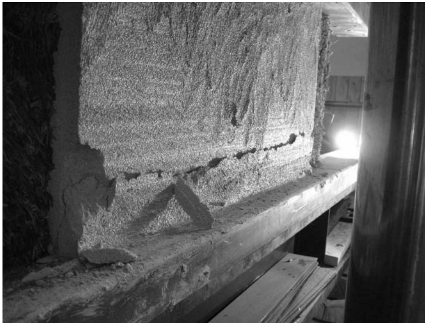
Figure 6.18b: Failure of Specimen C13
