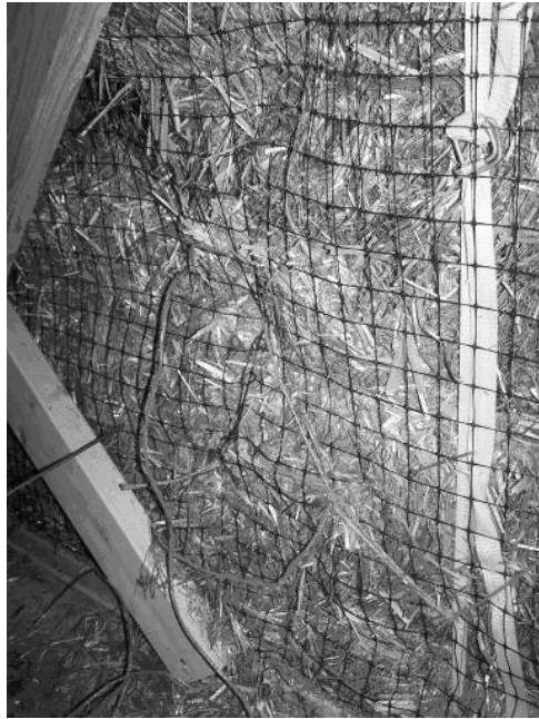
Figure 1.5: Mesh Applied to Straw Bale Wall
