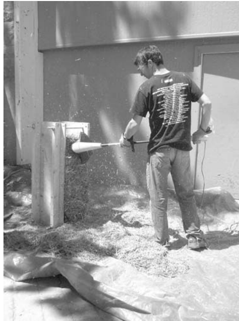
Figure 3.17: Trimming Straw Bale in Fabrication Jig
