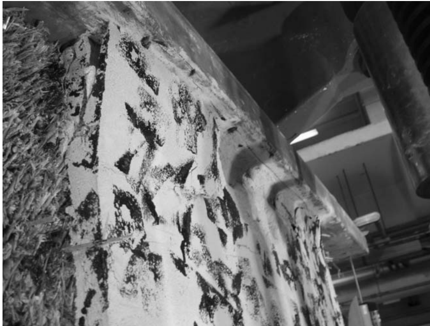
Figure 6.19b: Failure of Specimen C31
