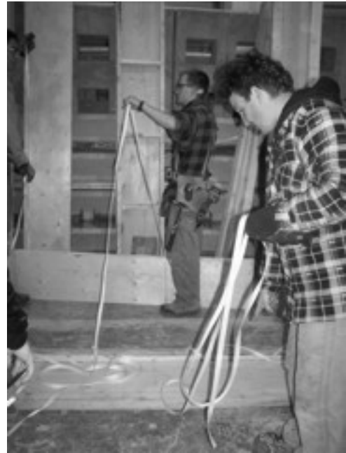
Figure 1.3: Strapping for Pre-Compression
