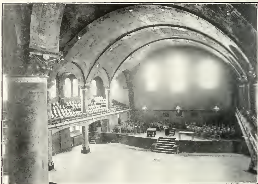
INTERIOR GRANT HALL.
