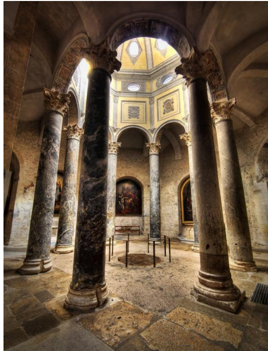
[Figure 39] The Baptistery of Saint-Sauveur in Aix-En-Provence, late 5 th century. Buttressing added in the 11 th century, dome partially remodeled in 13 th century. Loas, “Provincial Baptisteries,” 244, fig. 52.
