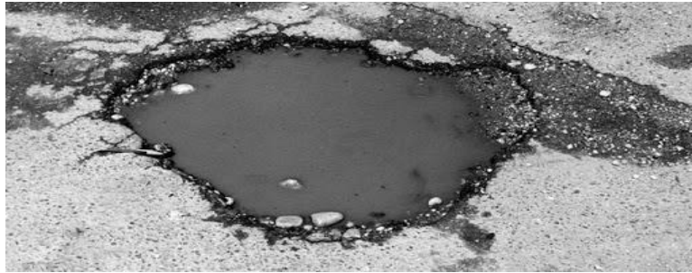
Figure 2.6: Moisture damage [31].
