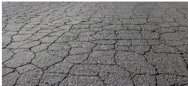
Figure 2.4: Fatigue cracking [26].
