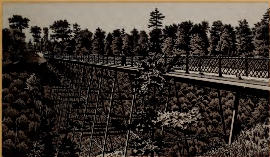
BRIDGE SPANNING, ROSEDALE RAVINE.
