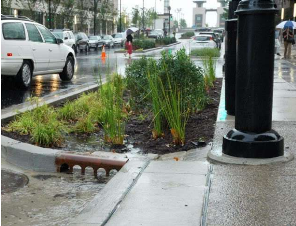
Figure 41: Traffic-calming curb bump-out in Pittsburg doubles as an enhanced stormwater catchment planter. Source: http://www.project15206.org/
