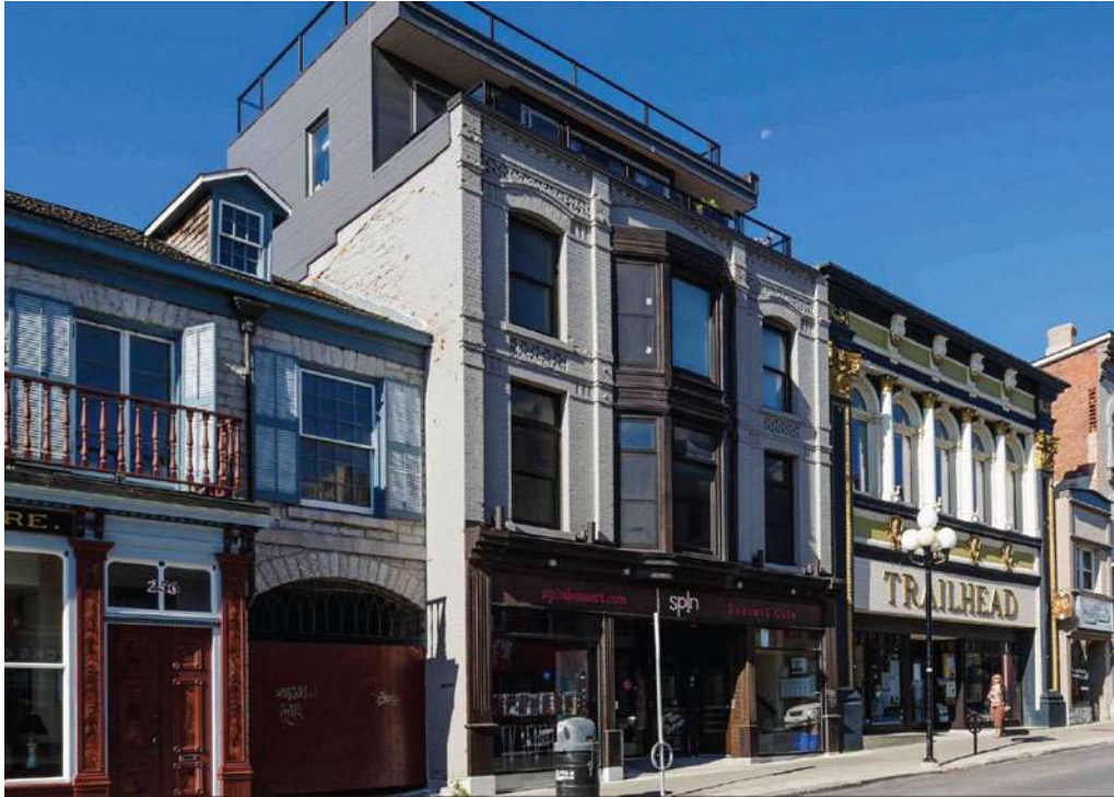
Figure 39: Infill development along Princess Street is modern in style but is set back from the street and creates an interesting building articulation along the streetscape.
