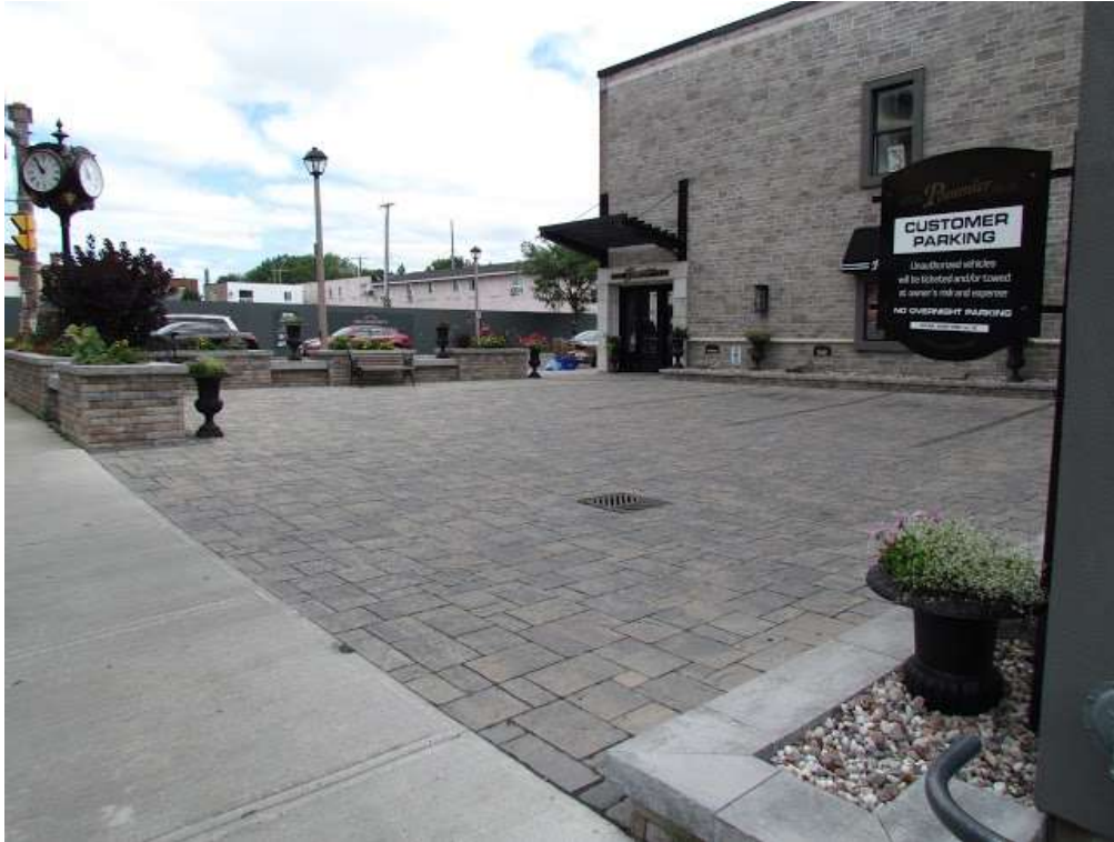
Figure 17: A corner parking lot at the corner of Pitt Street and Second Street in Cornwall has been enhanced with quality paving materials and planters, however, it is not appropriate for such a busy intersection.
