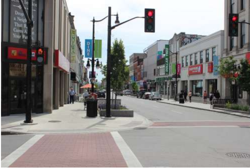
Figure 25: Street trees, furniture and lighting are strategically placed along the Princess Street ROW.
